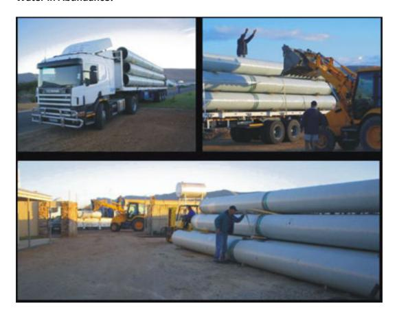
In order to pump more water to Bergsig farm and save electricity at the same time, a new 700mm pipeline of  $\pm$  450 metres in length was required. This new pipe was routed from the Sea View pumphouse, across the farm and all the way around the perimeter of Bergsig. The project was planned and executed in its entirety by Abagold personnel under the professional guidance of Abagold's engineer, Christiaan de Wet.
