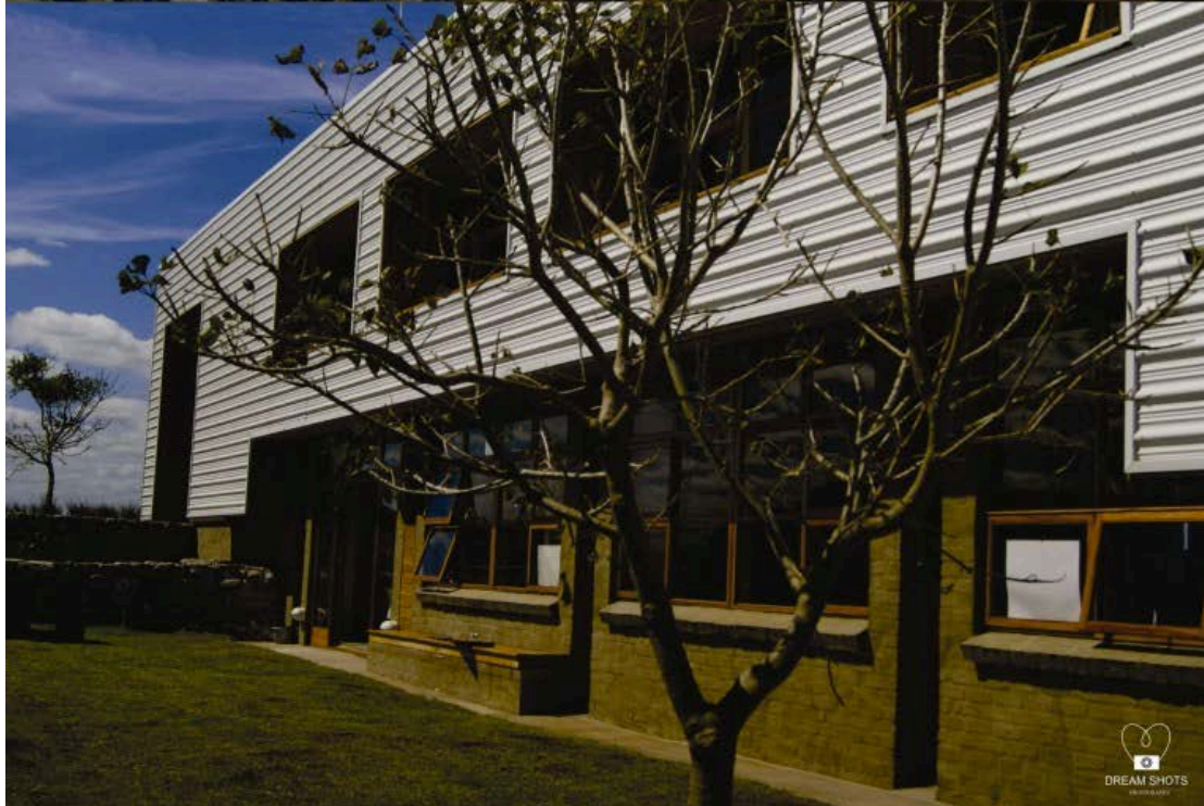
The side view of the offices showing the tearoom and garden area.
