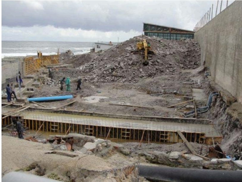
The dam under construction
