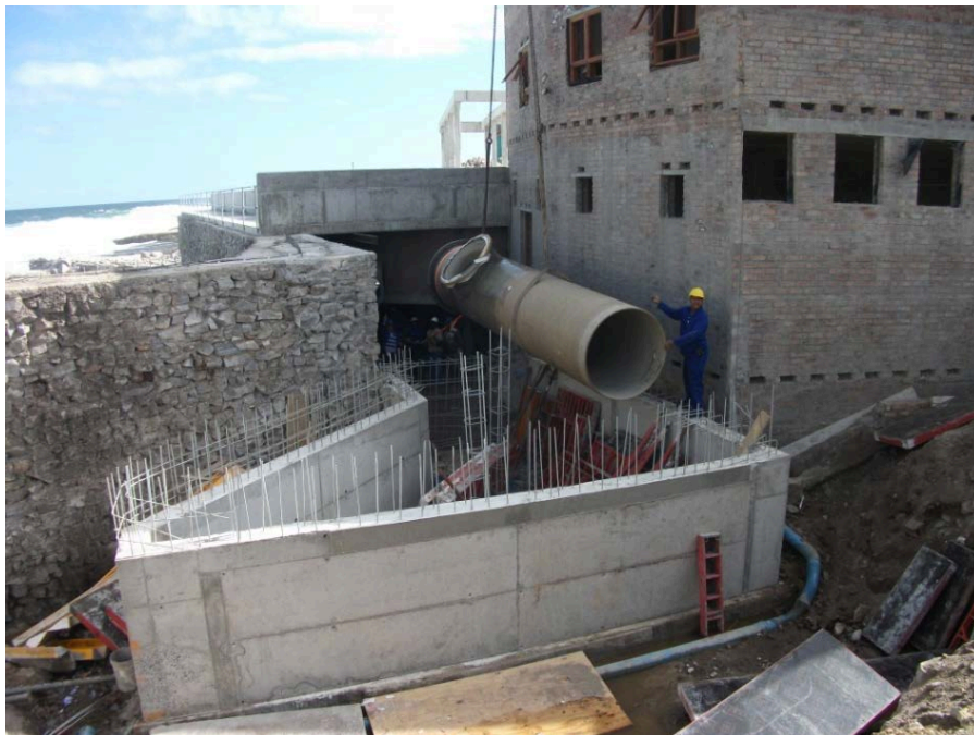
1200mm Pipes being installed
