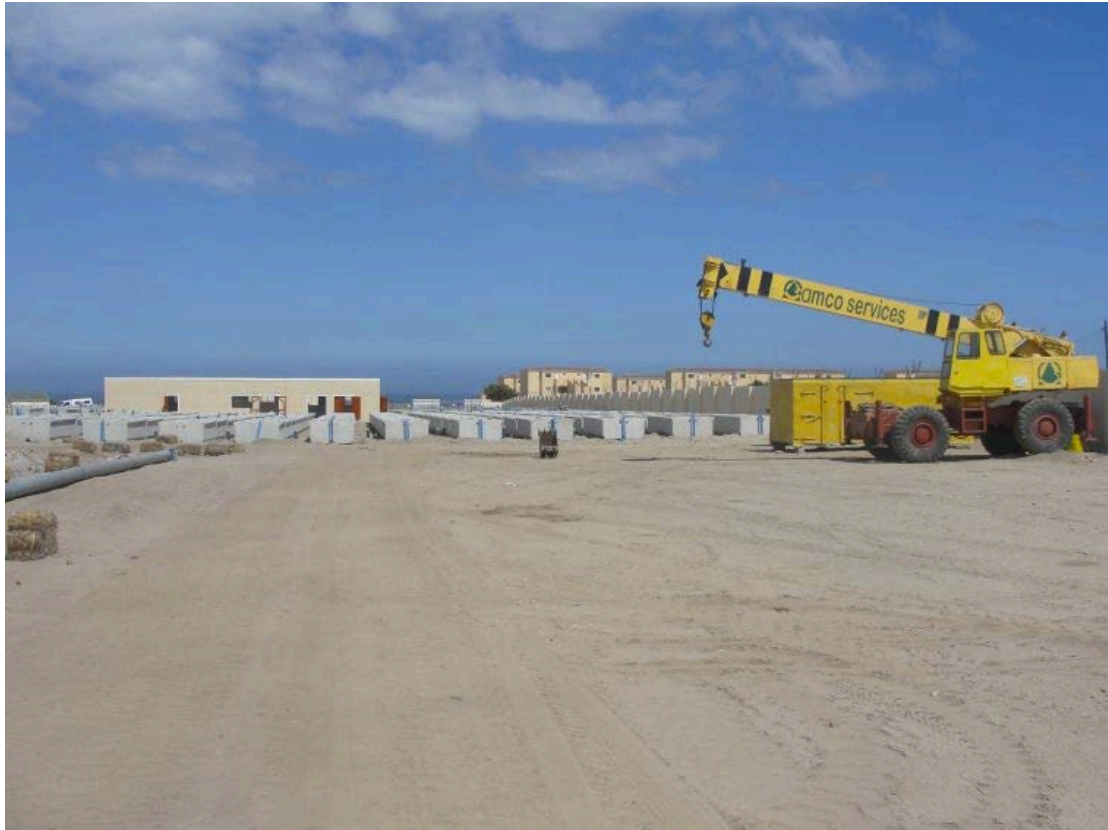
The first tanks installed
