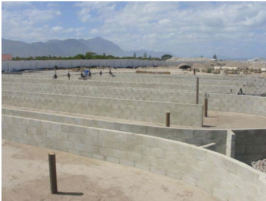
The newly built sea weed tanks
