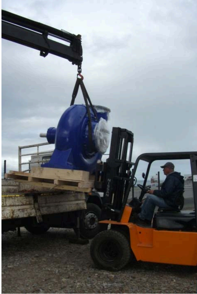
The pumps being offloaded
