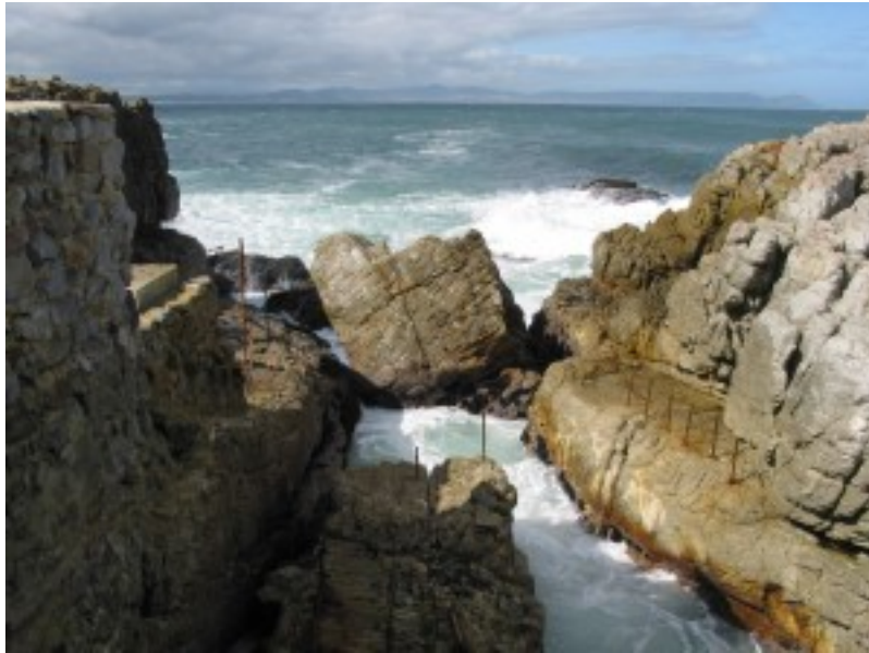
Widening of the canal progressing
