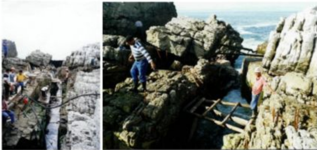
Constructing the inlet canal to the sump
