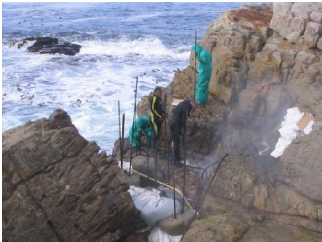
Preparations for the next set of concrete filled bags
