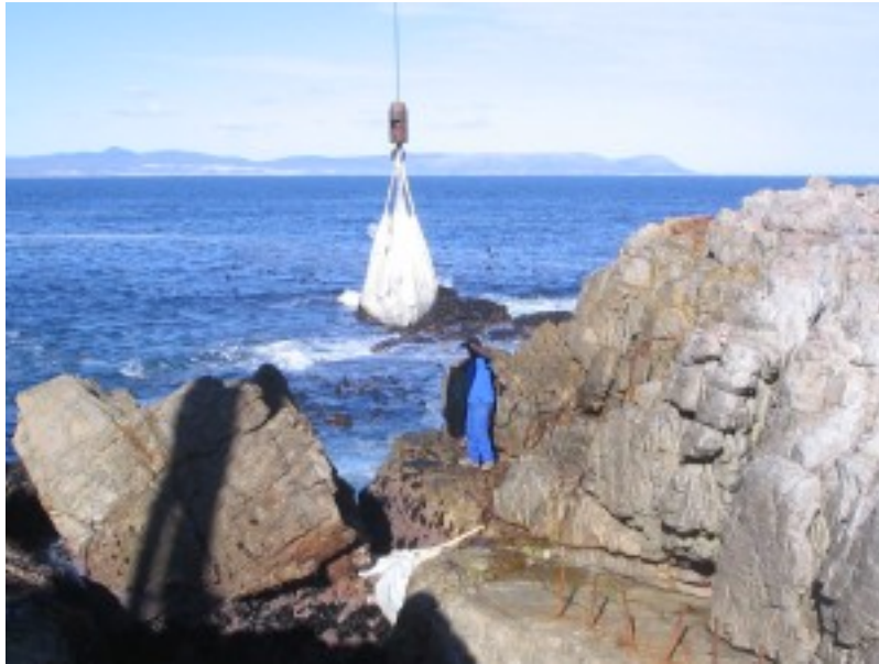
A bag filled with concrete being positioned
