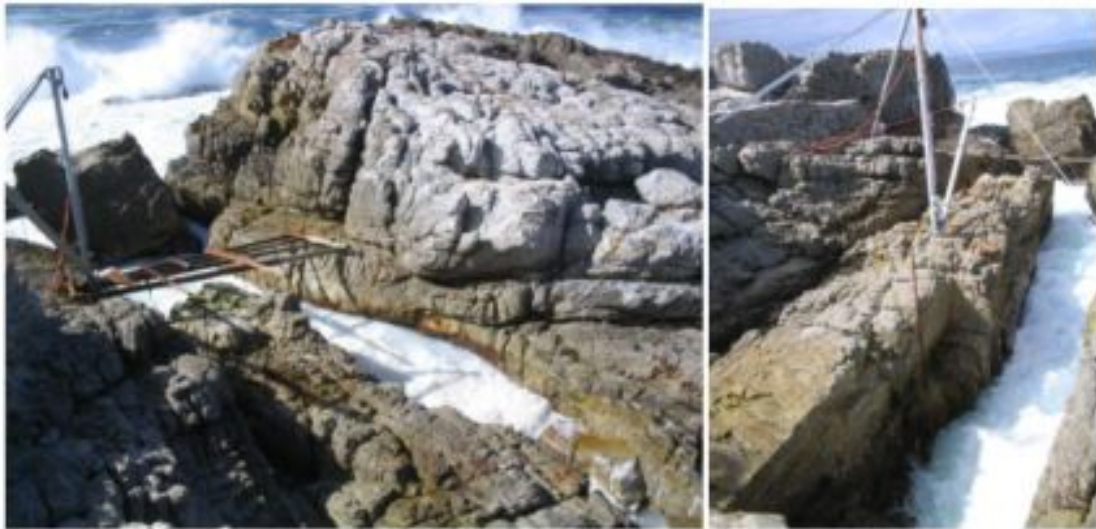
Widening of the inlet canal
