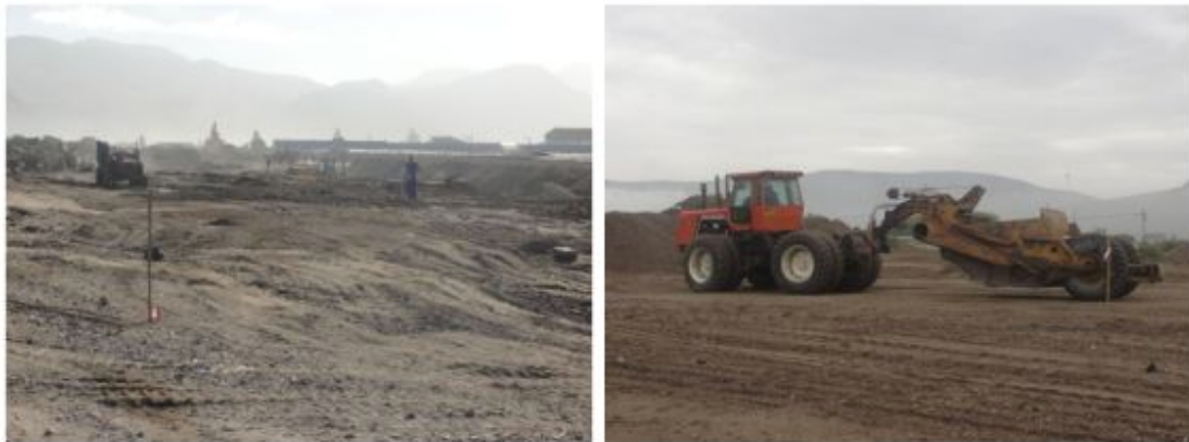
A section of the platform being levelled
