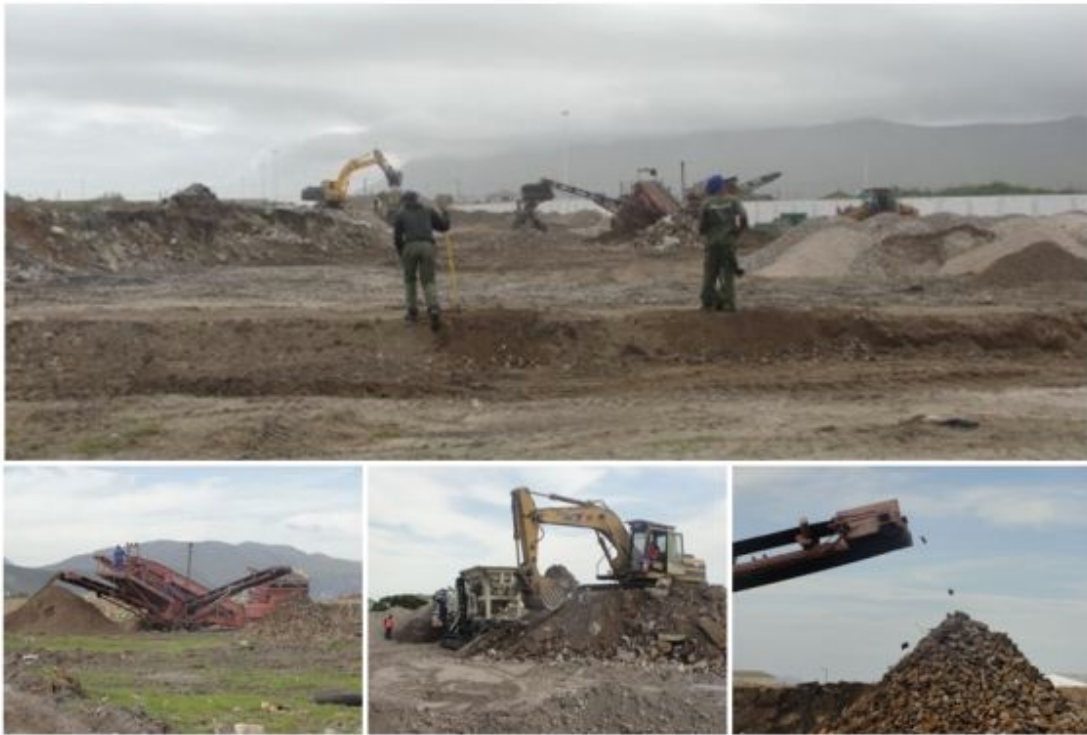
The Stone Crusher and Screen creating fill material of high quality
