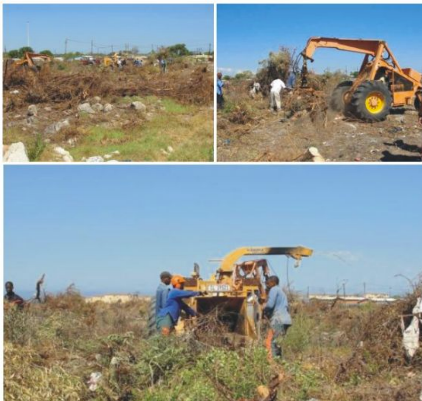
An Environmental Impact Assessment was completed and after receiving the "go-ahead" the teams started clearing the property.
