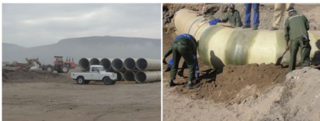
The 1200mm Main seawater pipes made from GRP
